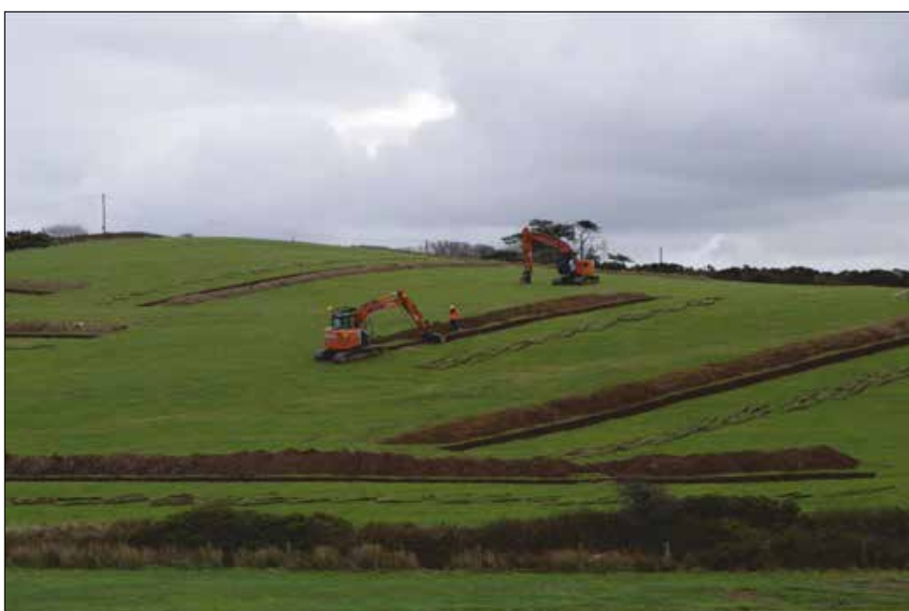
Plate 2: Soil stripping in Field A7
